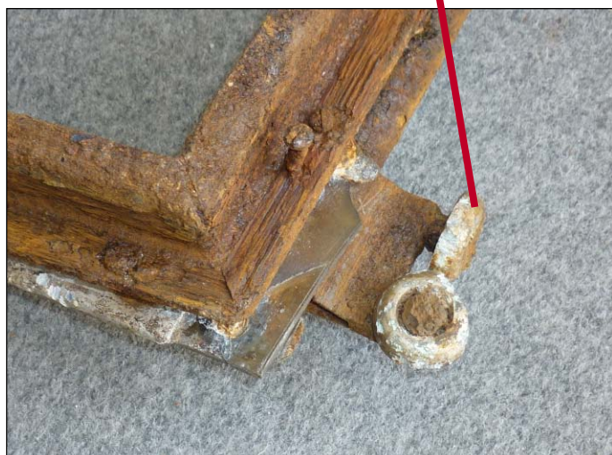
Detail view of the forward / bottom corner of the window – viewed from the outside. The arrow is pointing to a travel mechanism for pulling of the canopy. Note the remains of the Perspex and trace of wood on the metal frame.
