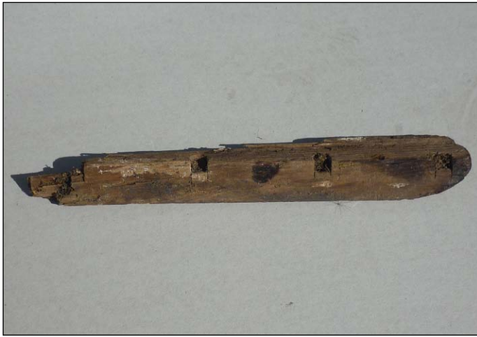
Portion of the armored glass wooden framing. Note the depressions in which the screws were countersunk, joining the metal frame with the canopy construction.
